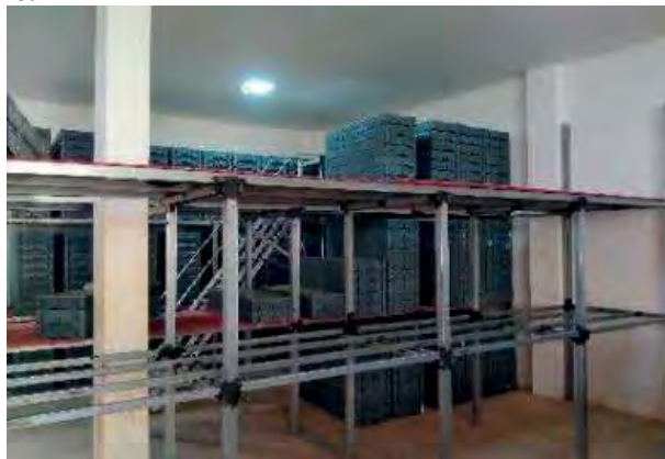
Figure 8. Sonic drill core storage galpao.
