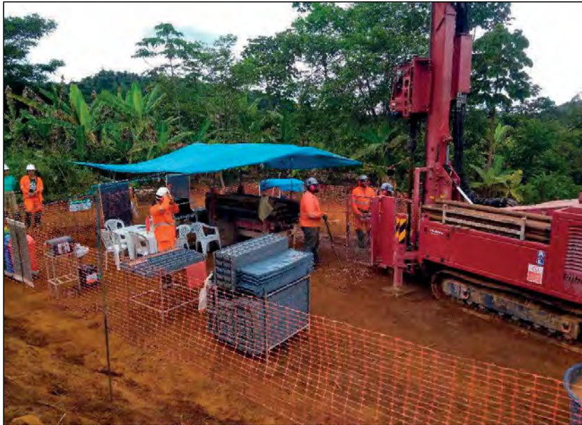
Figure 32 : Sonic drill rig set up Source: CSA Global 2023
