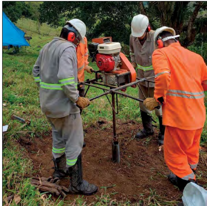
Figure 12. Mechanical auger in operation Source: BRE 2023
