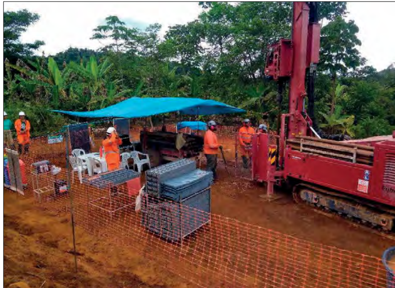
Figure 13. Sonic drill rig in operation Source: CSA 2023
